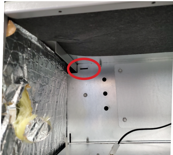
Figure 12. Notch for Control Panel Relocation
